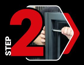
Wind out the adjustable anchors to get the frame held in position.
