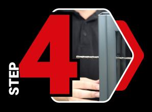
Drill though the centre of the adjustable anchors and use the same holes to insert the fasteners.
